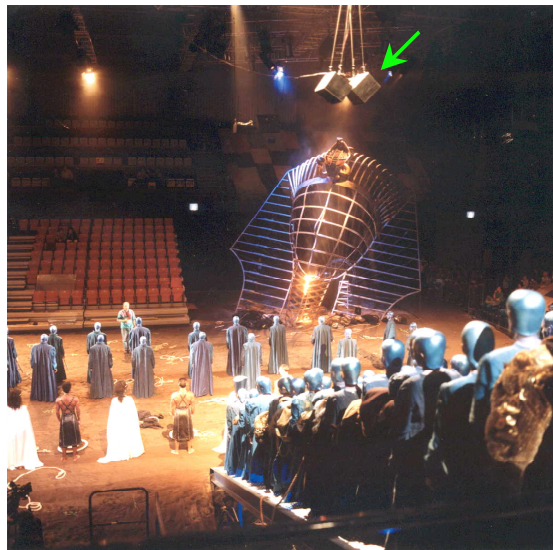
Figure 2: Example of actual loudspeaker location during the Aïda opera in Amsterdam, The Netherlands. The arrow points at the loudspeakers that provide lateral energy for two different subsections.
